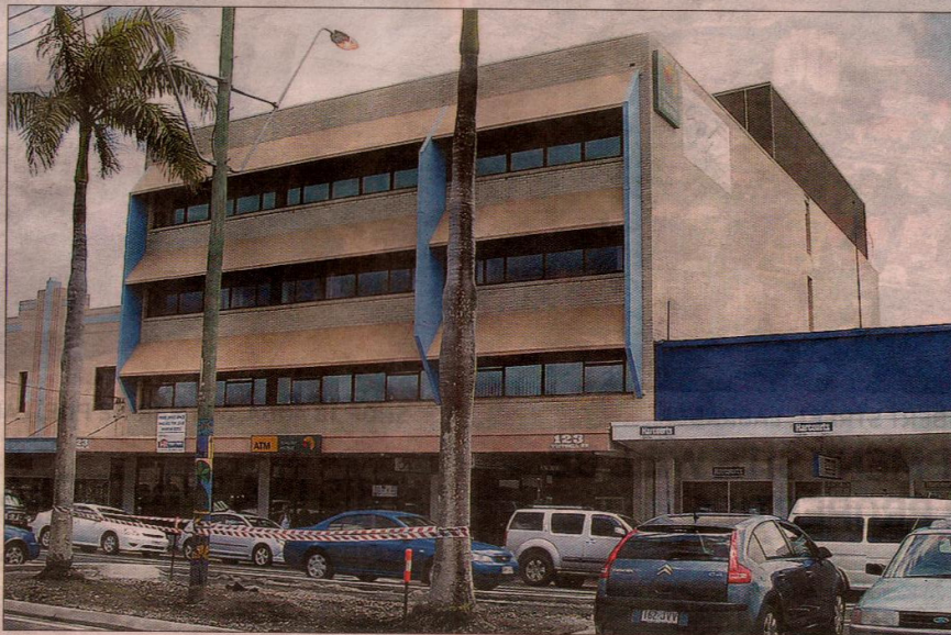
123 Victoria Street... one of two Mackay business district buildings bought for $7.5 million by Gold Coast interests and earmarked for makeovers in the next five years
